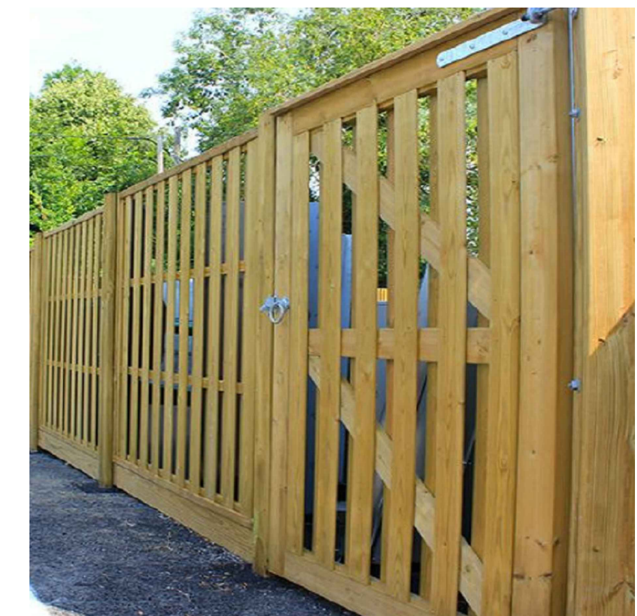
HIT & MISS TIMBER FENCING TO SPRINKLER TANK COMPOUND
